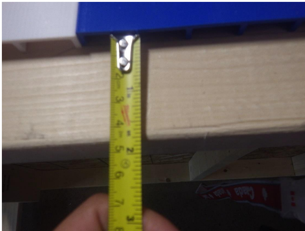
Photograph 6: Standard location of Fortress. 1 \frac{3}{8} " – 1 \frac{3}{4} " from inside
