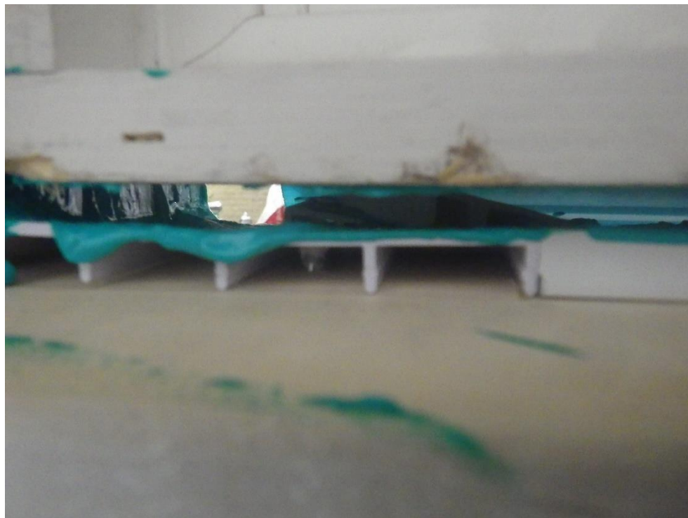
Photograph 10: Specimen A installation. Left corner (from indoor) Note gap between Fortress and window frame
