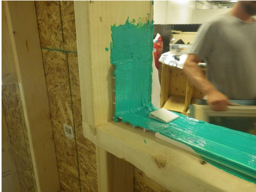
Photograph 7: Liquid sill membrane
