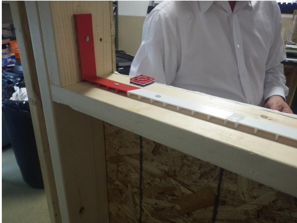
Photograph 5: Fortress center strip installation – 2 nd Generation
