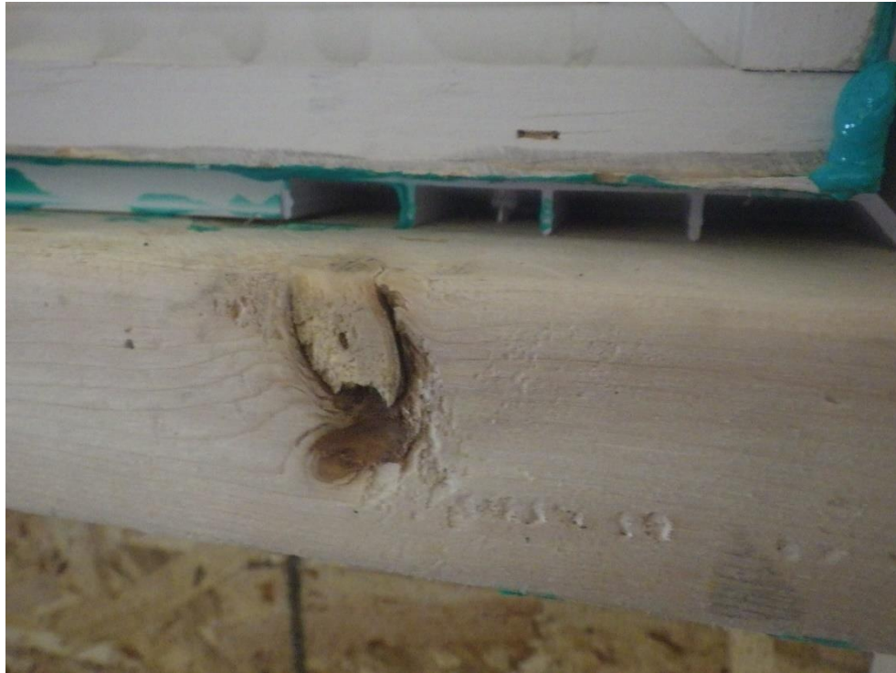
Photograph 11: Specimen A installation Right corner (from indoor)
