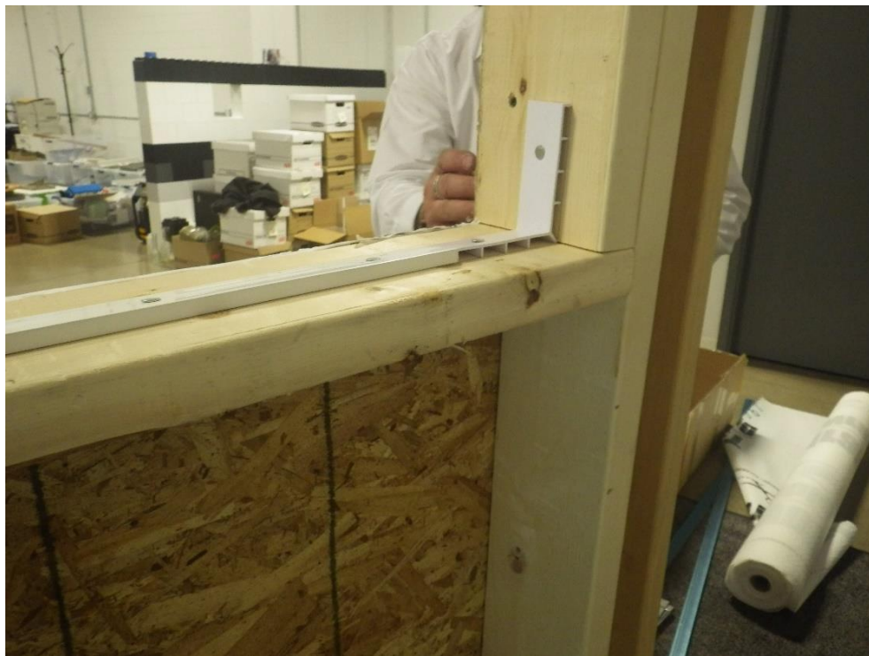
Photograph 4: Fortress center strip installation – 1 st Generation
