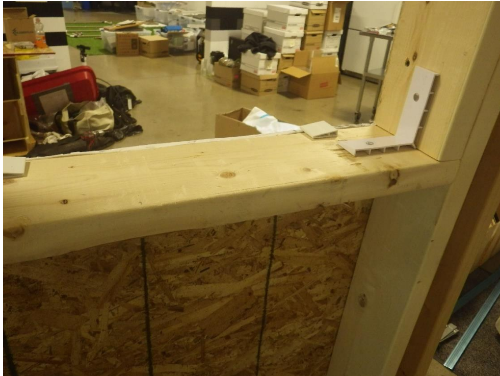
Photograph 3: Fortress corner installation
