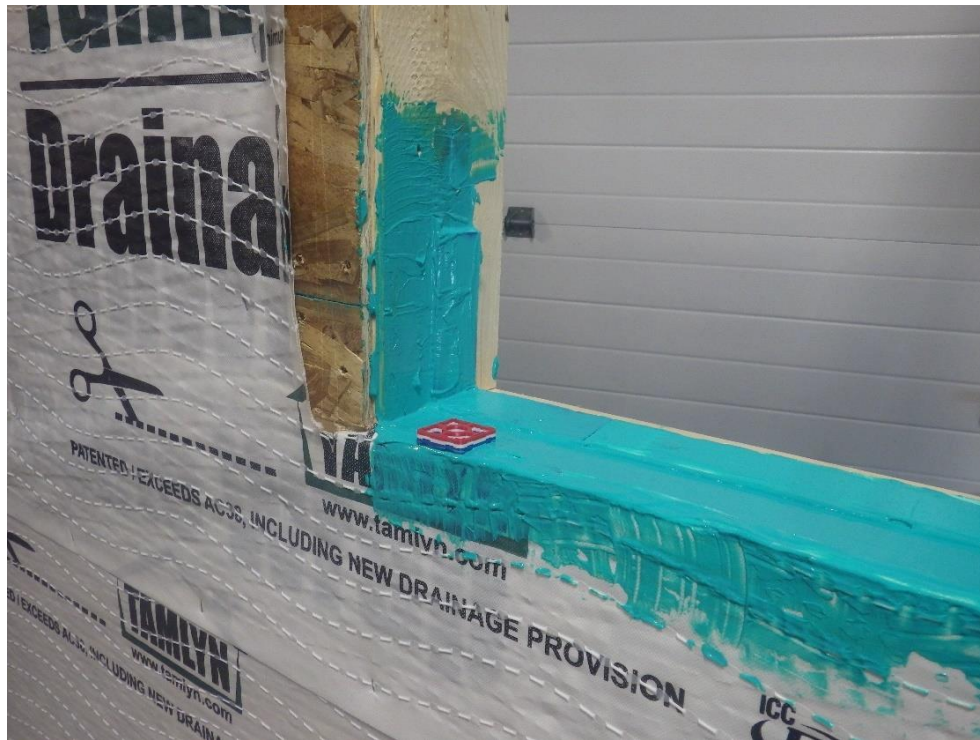
Photograph 9: Specimen B - Shimming
