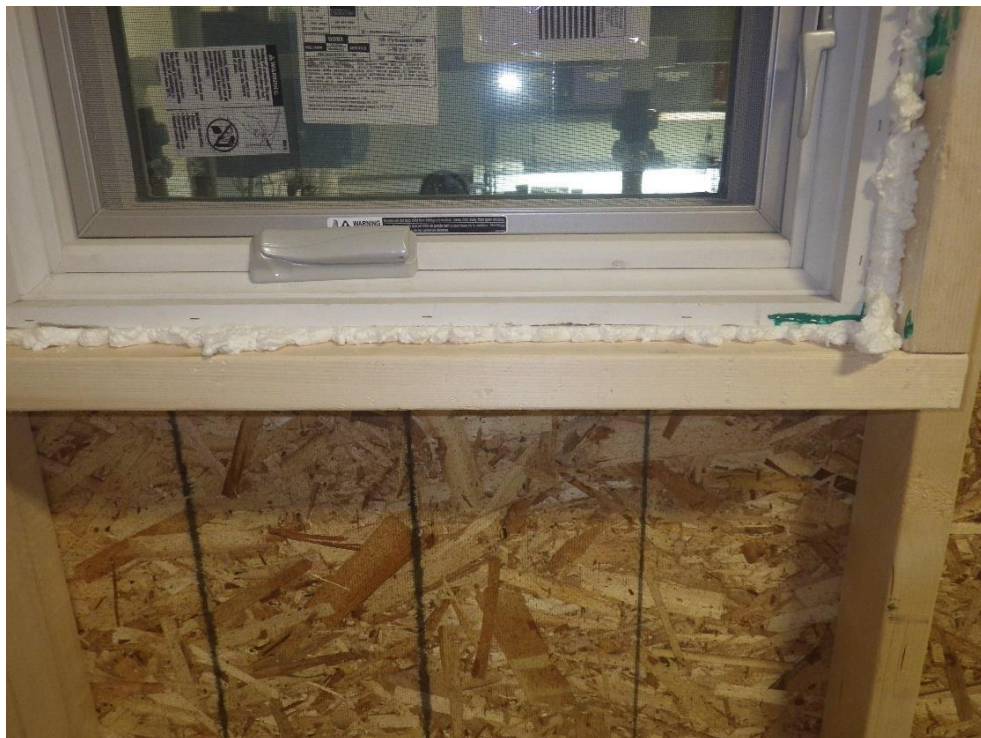
Photograph 18: Interior seal installation
