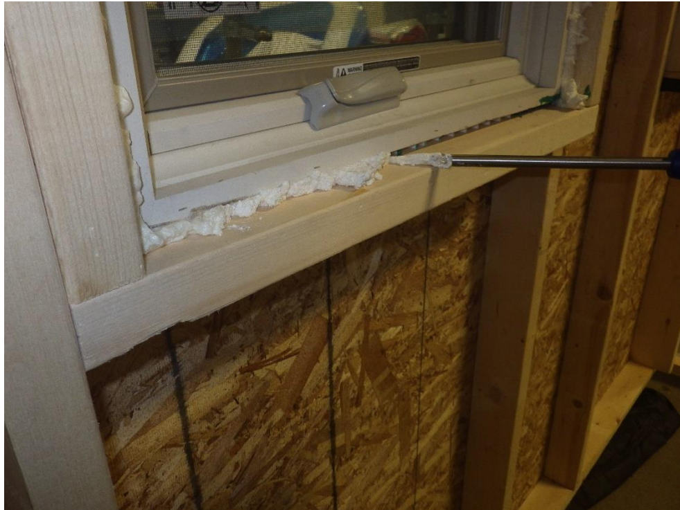
Photograph 17: Interior seal installation
